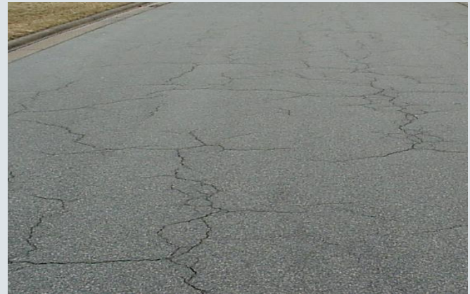
Block Cracking
