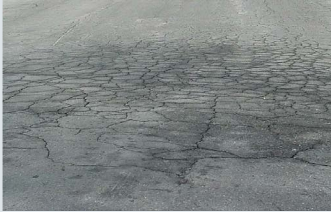
Alligator Cracking
