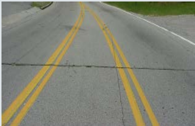
Reflective Cracking
