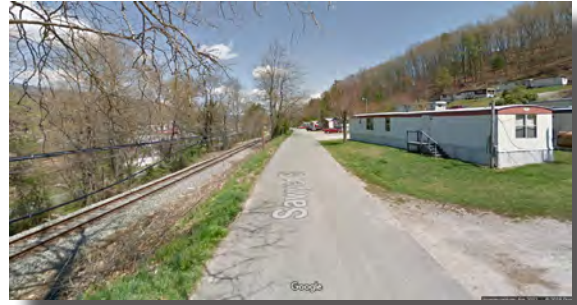
Potential for new development in the vicinity of Old Balsam Road south of the Smoky Mountain Expressway
