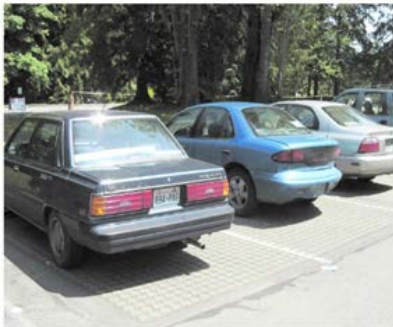
Pervious pavers and other pervious paving techniques allow stormwater to infiltrate
